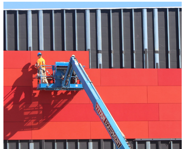
RevealShield SA Self-Adhered creates the desired black reveal and UV stability behind the open joint cladding.
